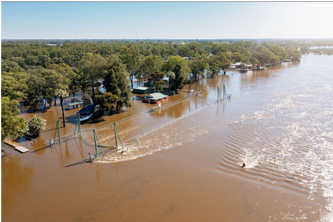
Lock 5 in Paringa was among the River Murray lock chambers closed throughout flooding down the river system.
