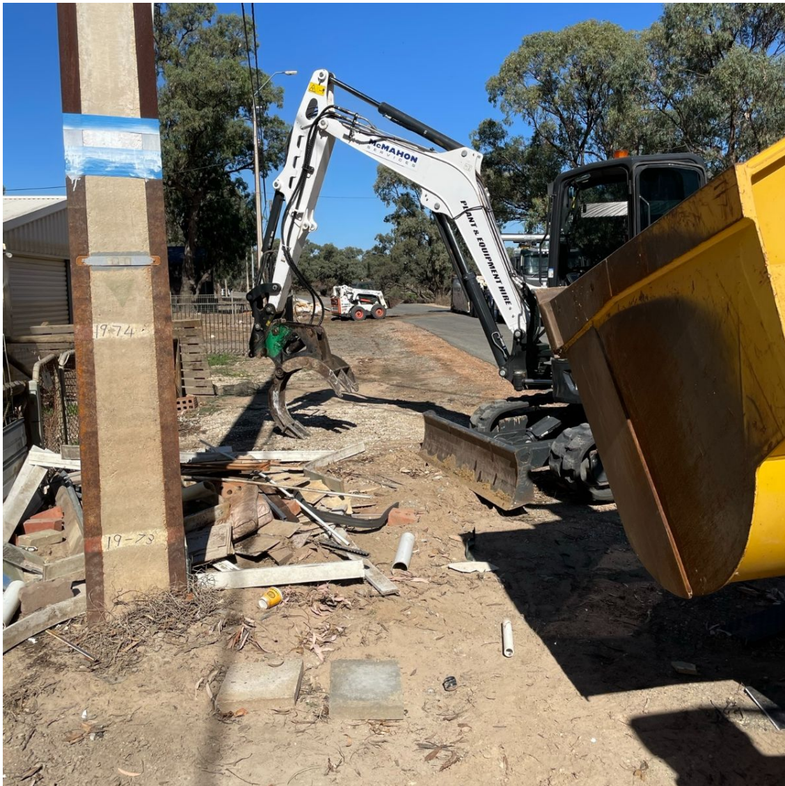
Clean-up efforts in Blanchetown earlier this week
